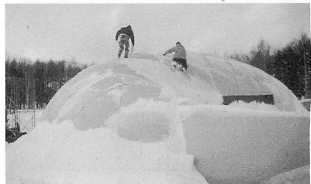
Fig. 5. Formwork for free-shape shell
