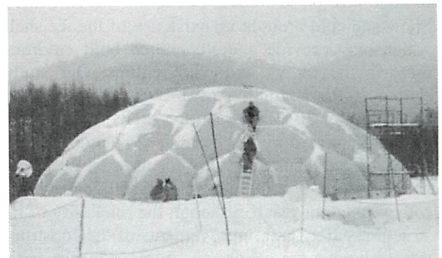
Fig. 11. Air-inflated membrane as formwork
