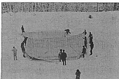
Fig.4. Placing membrane on the snow ground
