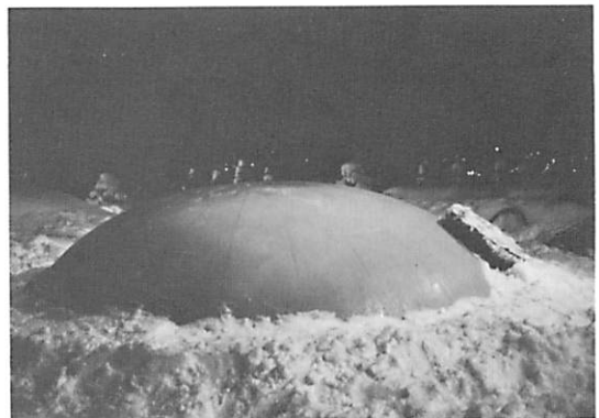
Fig. 3 Air-inflated membrane as tormwork
