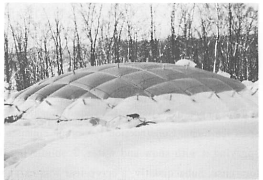
Fig. 2 Air-inflated membrane as formwork
