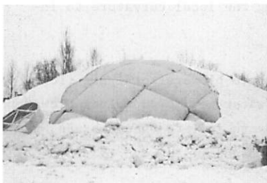
Fig.2 Removal of imperfect snow-ice at depression part
