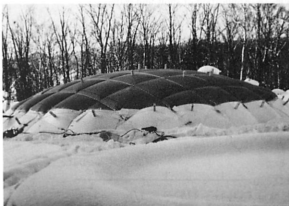
Fig. 13. Air-inflated membrane as formwork.
