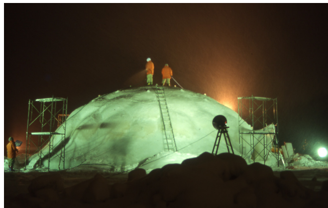
Fig.1 Spraying water on ice dome under construction
