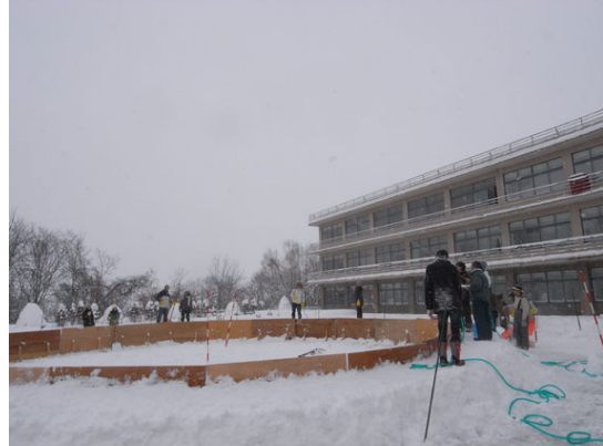
Fig. 9 Construction of snow-ice foundation ring
