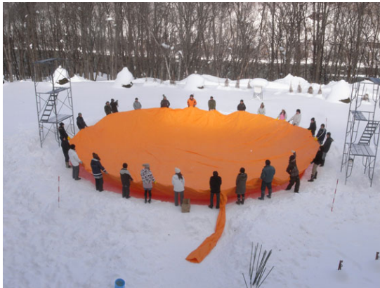
Fig. 10 Set up membrane bag
