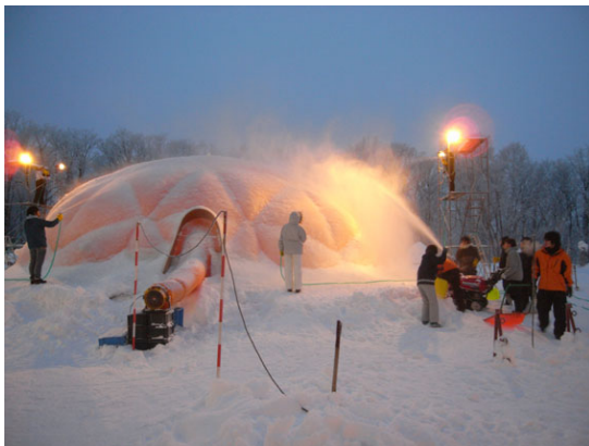
Fig. 12 Application of snow and water
