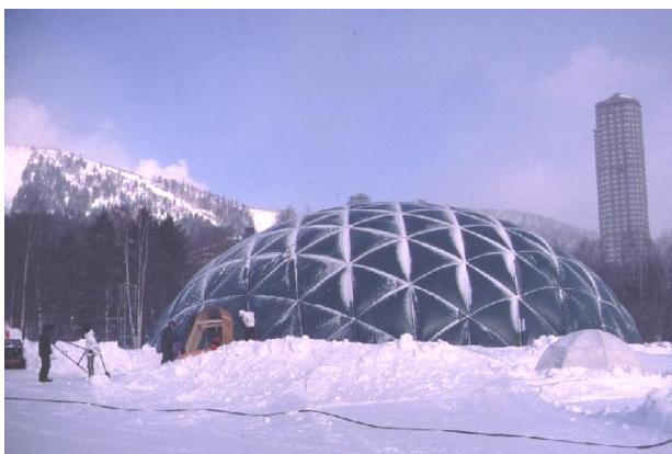
(c) Circular membrane bag (30m diameter) + Triangular pattern from Geodesic division [6]
