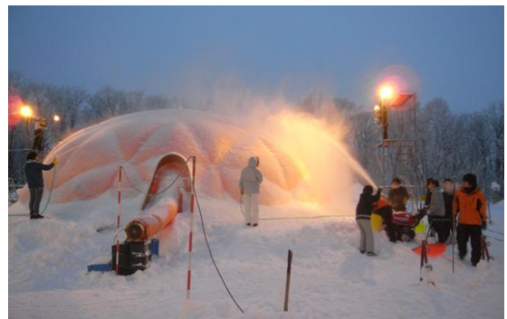
(c) Application of snow and water
