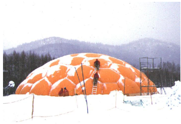
(b) Circular membrane bag (20m diameter) + Hexagonal and Pentagonal pattern from Geodesic [5]
