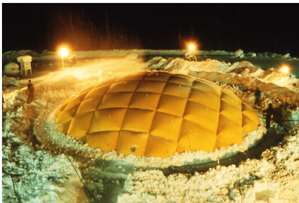
(a) Circular membrane bag (15m diameter) + Grid pattern [12]
