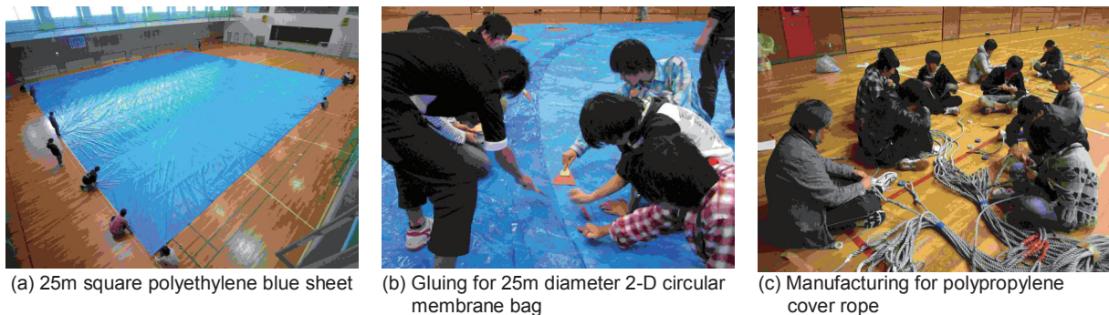
Fig. 7: Preparation for pneumatic formwork (IPP2012)
