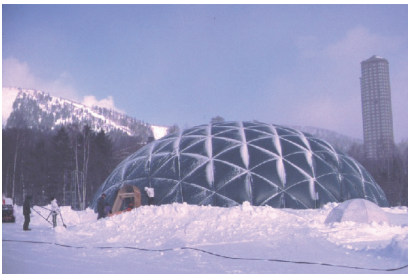
(c) Circular membrane bag (30m diameter) + Triangular pattern from Geodesic division[12]
