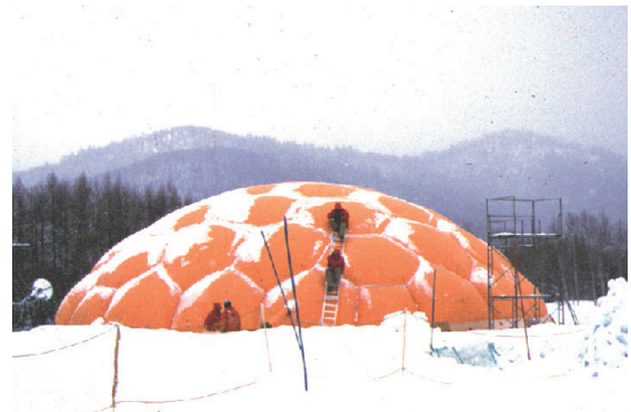
(b) Circular membrane bag (20m diameter) + Hexagonal and Pentagonal pattern from Geodesic[11]
