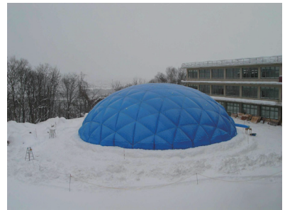
(c) 3-D air inflated formwork
