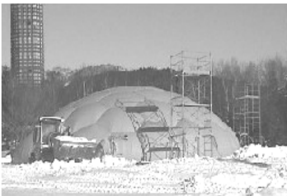
Figure 8. Air-inflated membrane as formwork.
