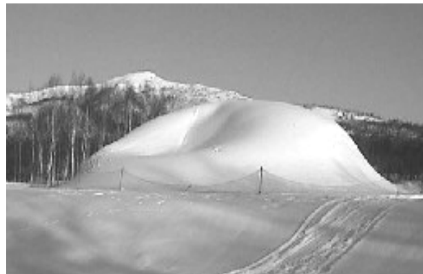
Figure 12. Large deformation right before collapse.
