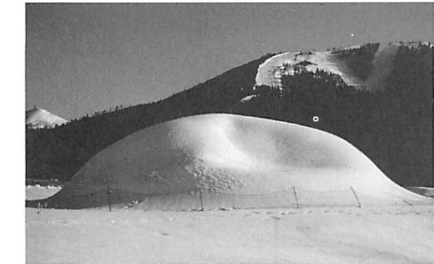
Fig. 11 Large deformation right before collapse
