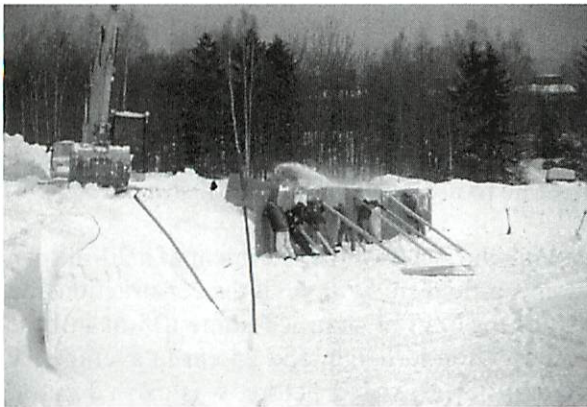
Fig. 1. Construction of snow-ice foundation ring
