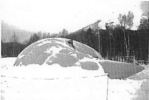
Fig.3 Formwork for free-shape shell
